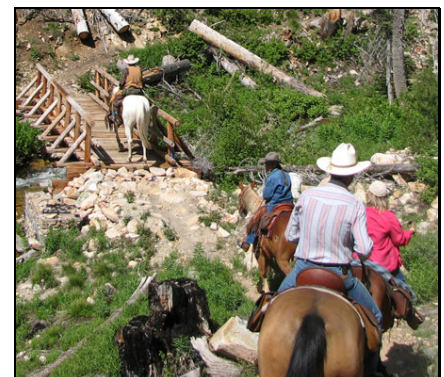
Gates Creek Bridge
