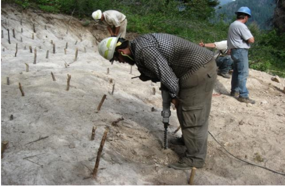
Blasting work with IDPR
